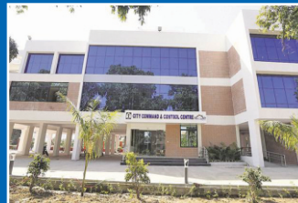
City Command Centre Vadodara
